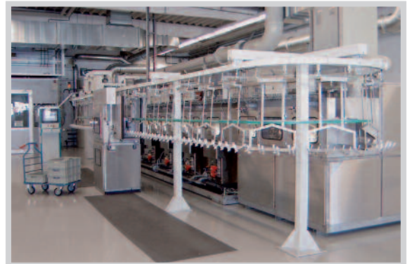
Pass-through spray facility with suspension conveyor
