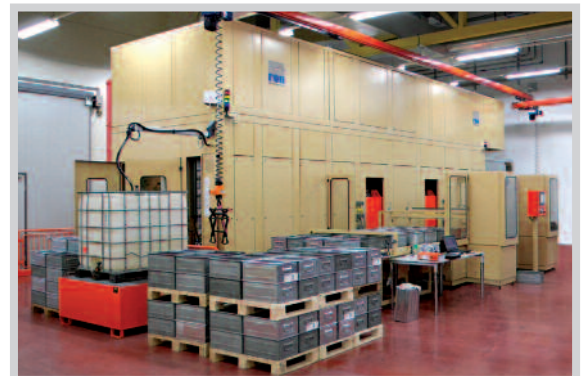
Special facility with a throughput of up to 75 baskets an hour
